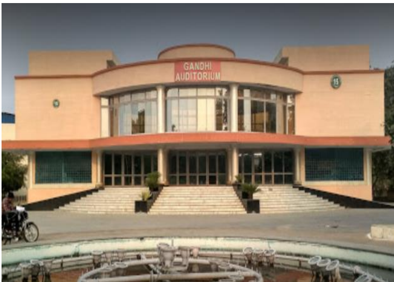
AUDITORIUM AT BUNDELKHAND UNIVERSITY, JHANSI
